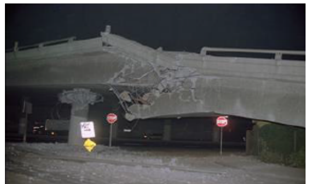
Figure 1: Bridge collapse in Northridge.
