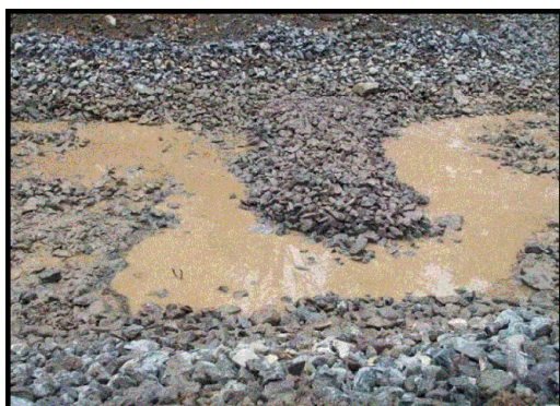
Figure 7: Physical hydrological features under construction in Cell 1 on October, 2010.
